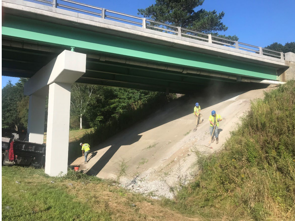
Clean up at Wilson Road Bridge.
