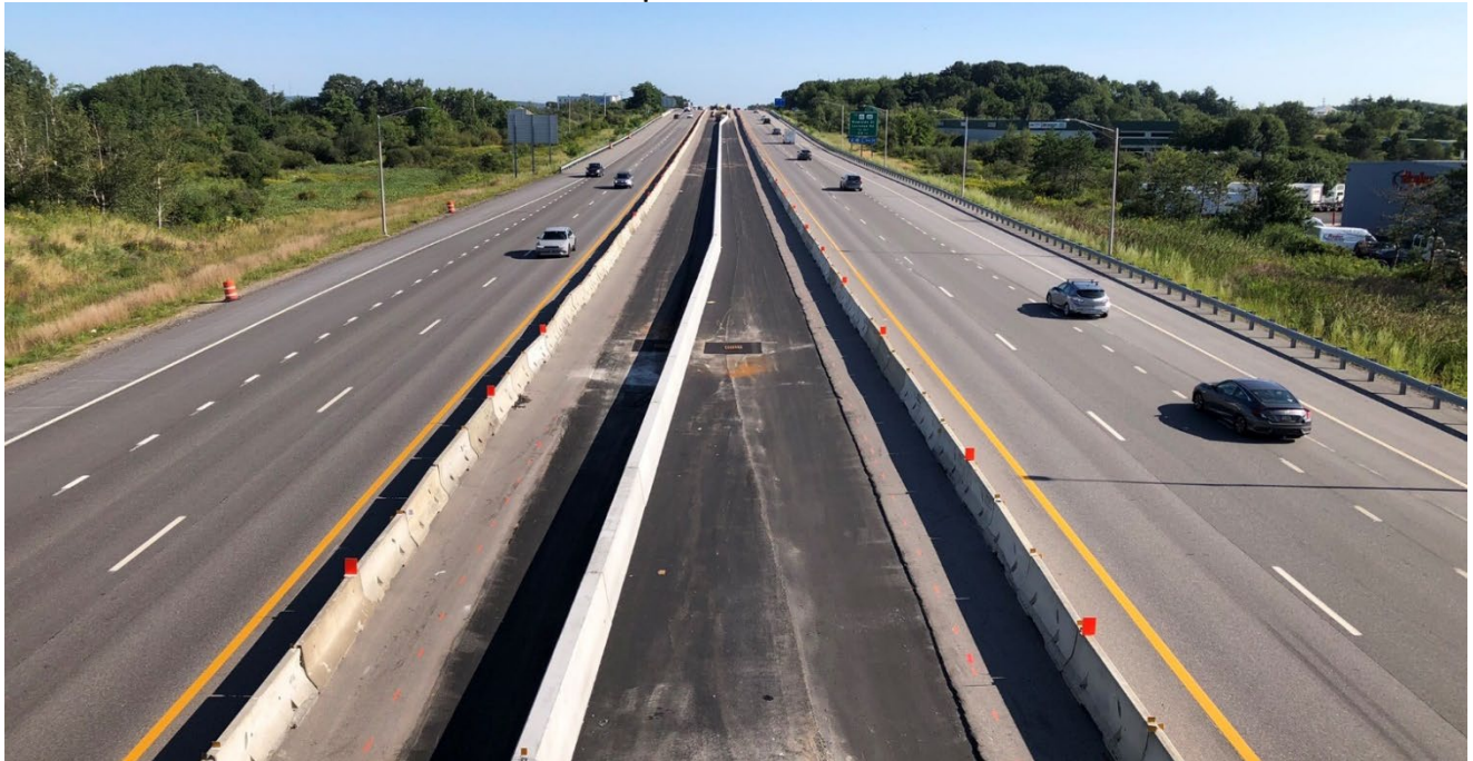
Median construction completed to Maine Central Railroad
