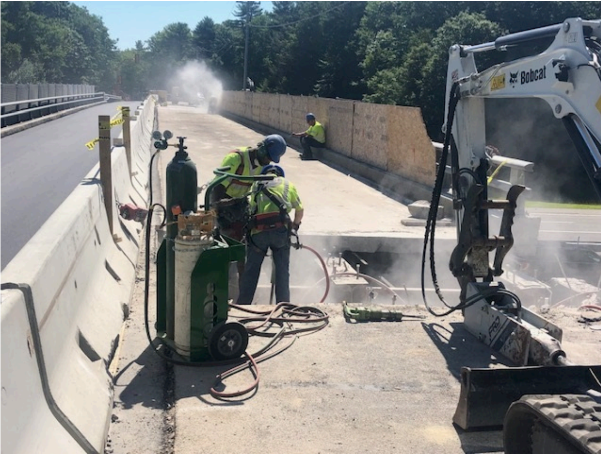
Working at Mountain Road backwall
