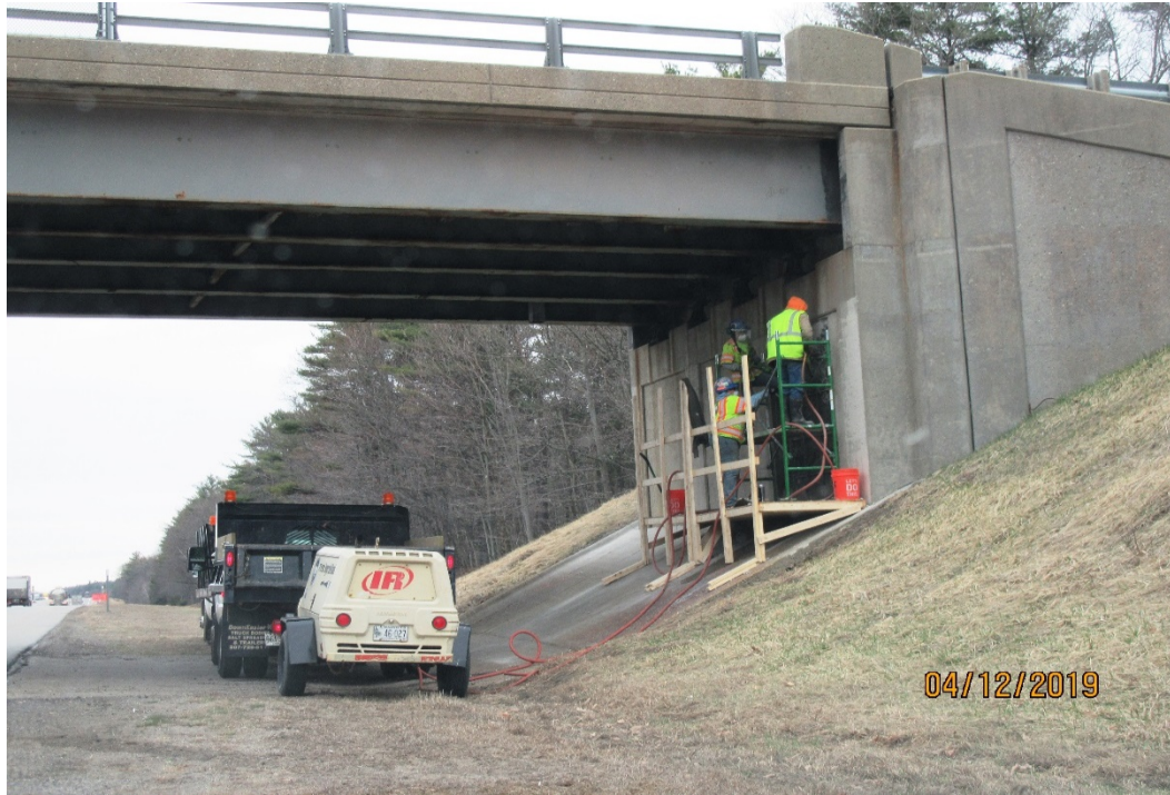
Mountain Road North Bound Abutment
