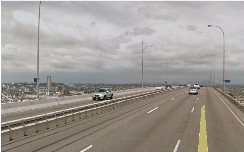
Figure 3 – San Diego-Coronado Bridge
