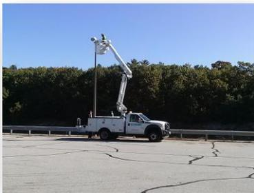
In 2016 approximately 205 existing highway and site lighting luminaires were replaced with LED luminaires at Maine Turnpike entering and existing ramps, toll plazas, service plazas, and maintenance yards. The work included verifying existing luminaire and circuit voltages, furnishing and installing replacement LED luminaires and furnishing and installing pole breakaway splice kits, if non-existent.
