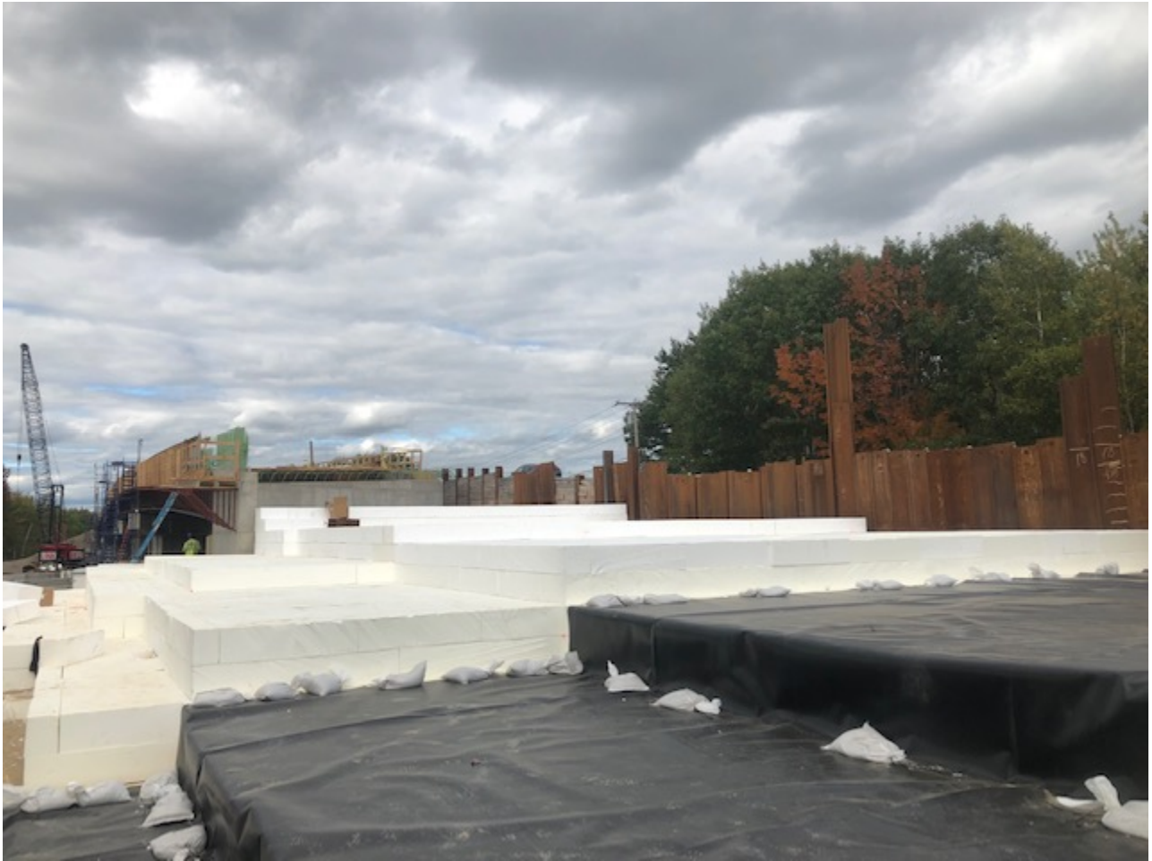
Geofoam light weight fill southern approach
