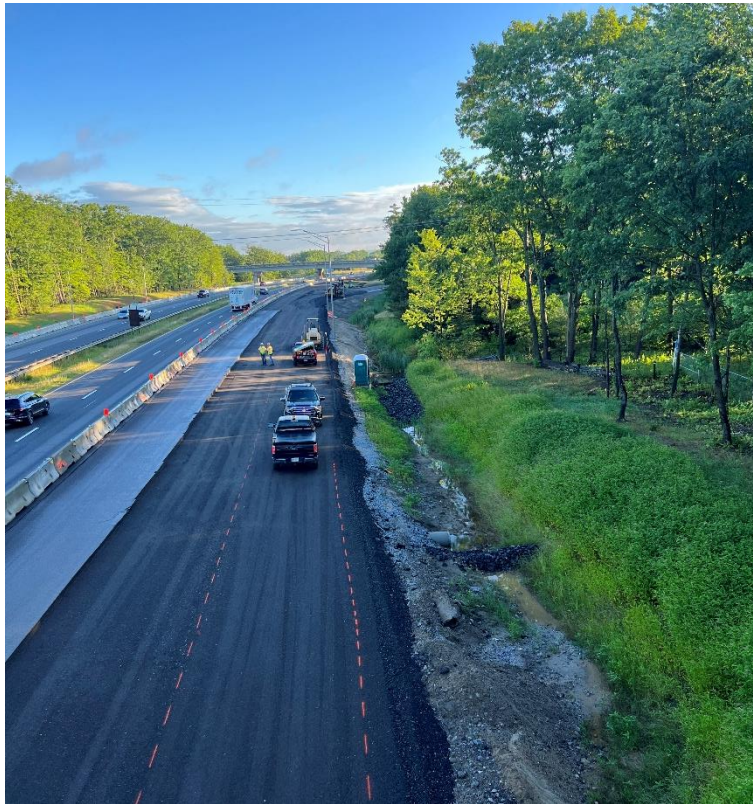
Grading mainline during the Exit 47 Shutdown
