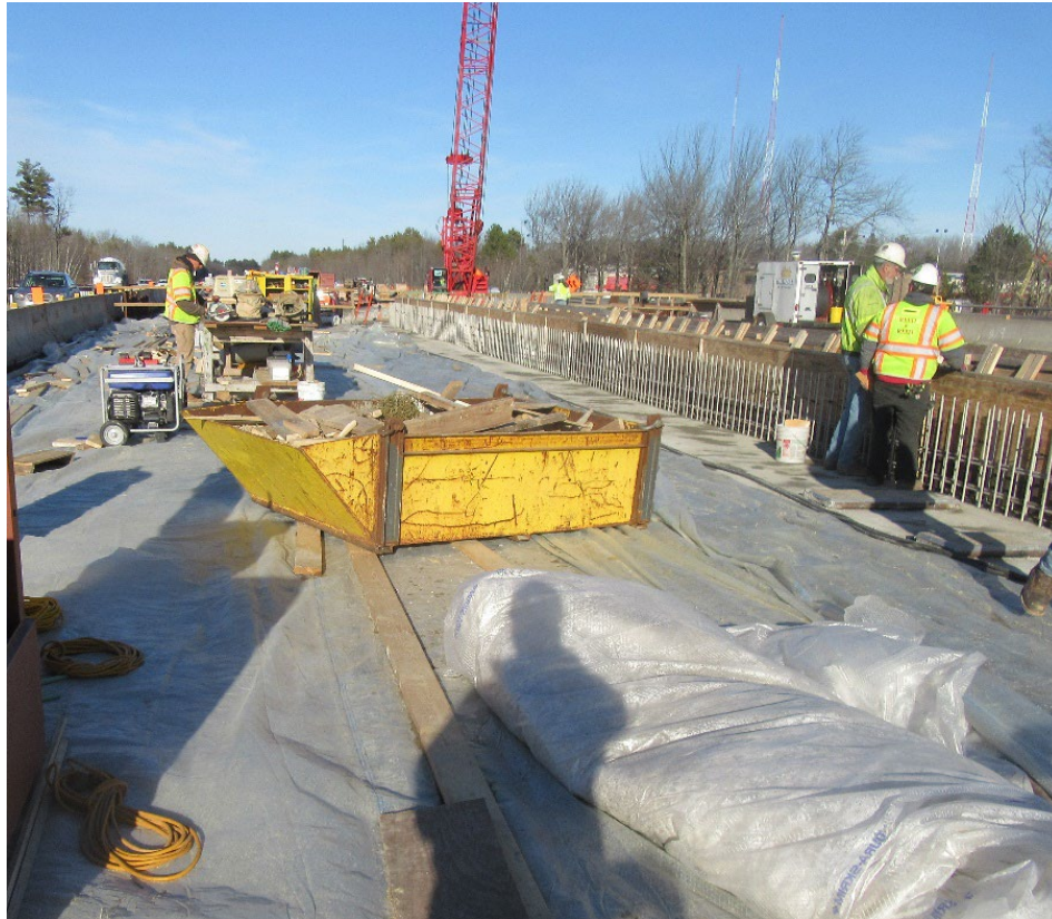
Southbound bridge deck
