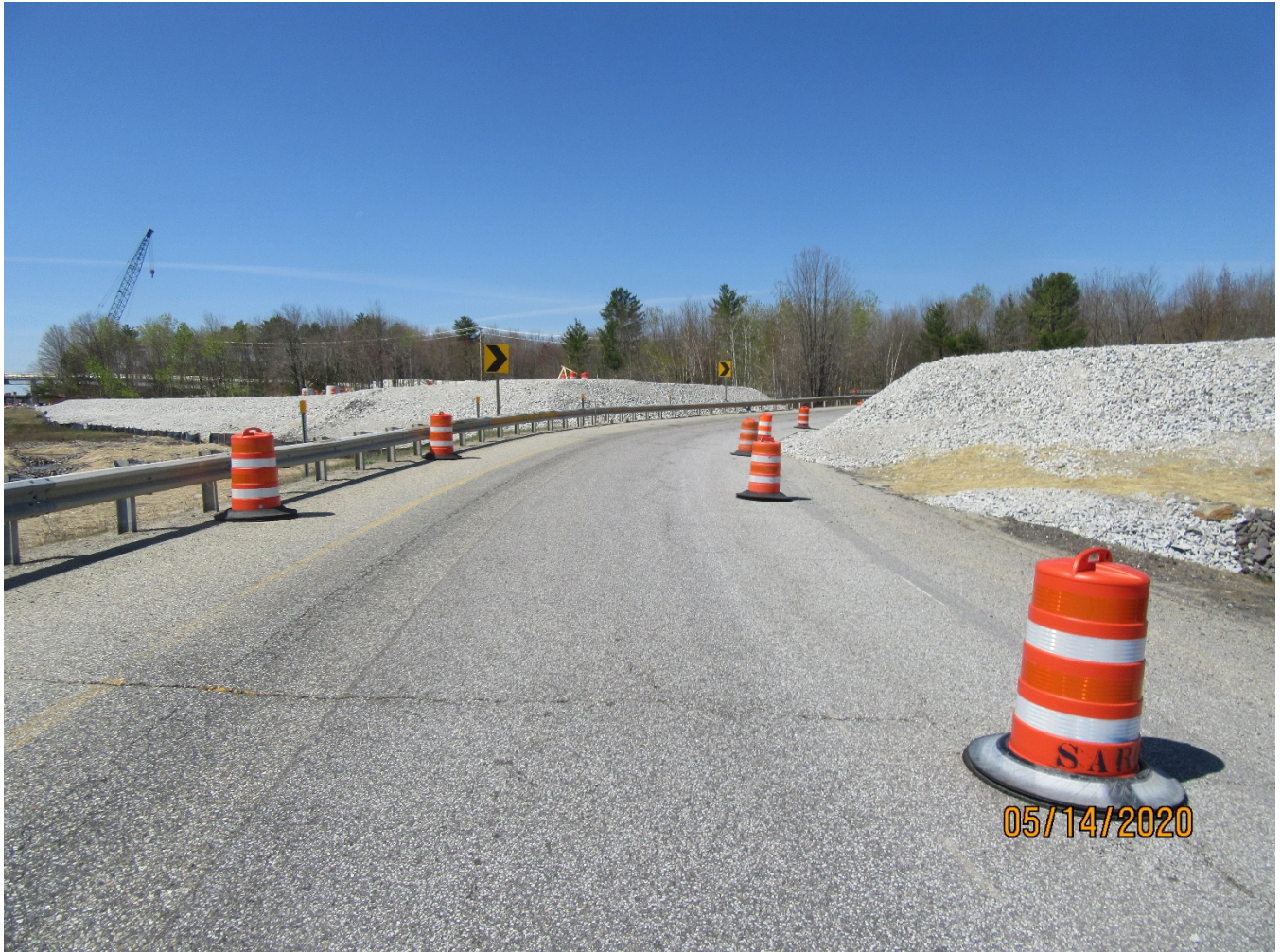
Preload either side of the Exit 45 southbound off-ramp
