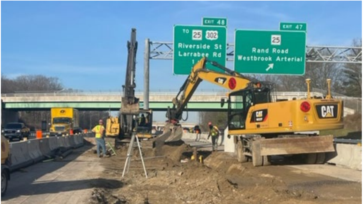
Installing Median Drainage at Exit 47 looking north
