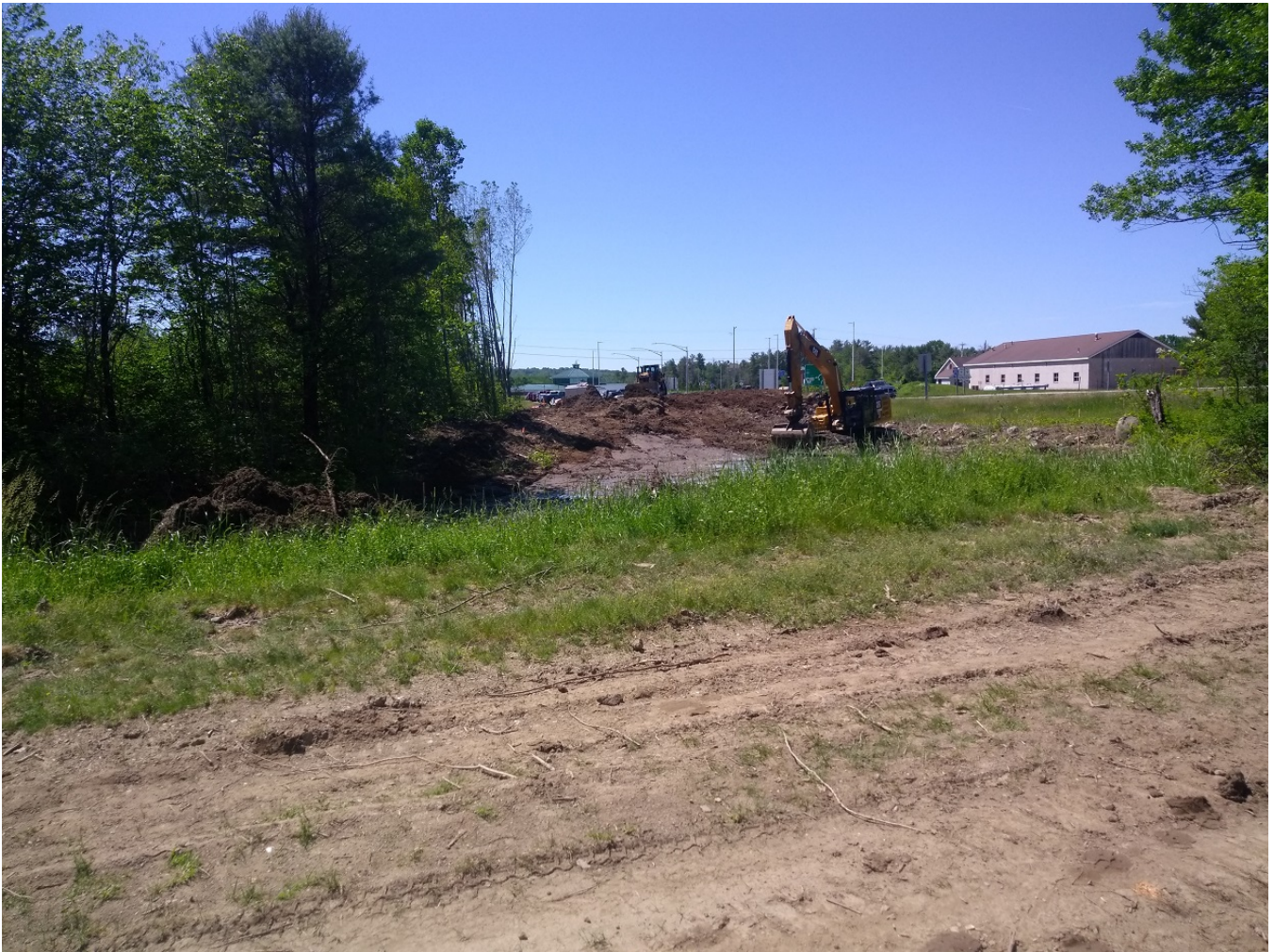
Grubbing topsoil for the new access road
