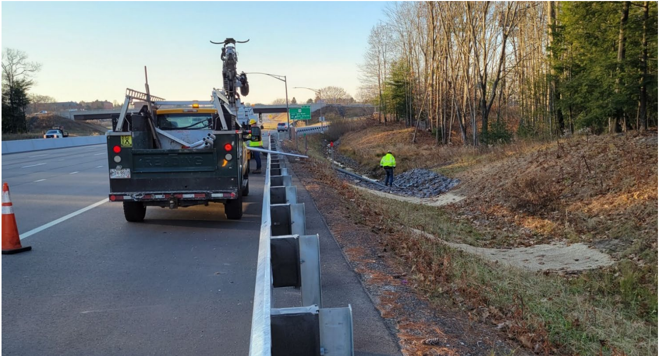
Upgrading light poles at Exit 48 SB off ramp
