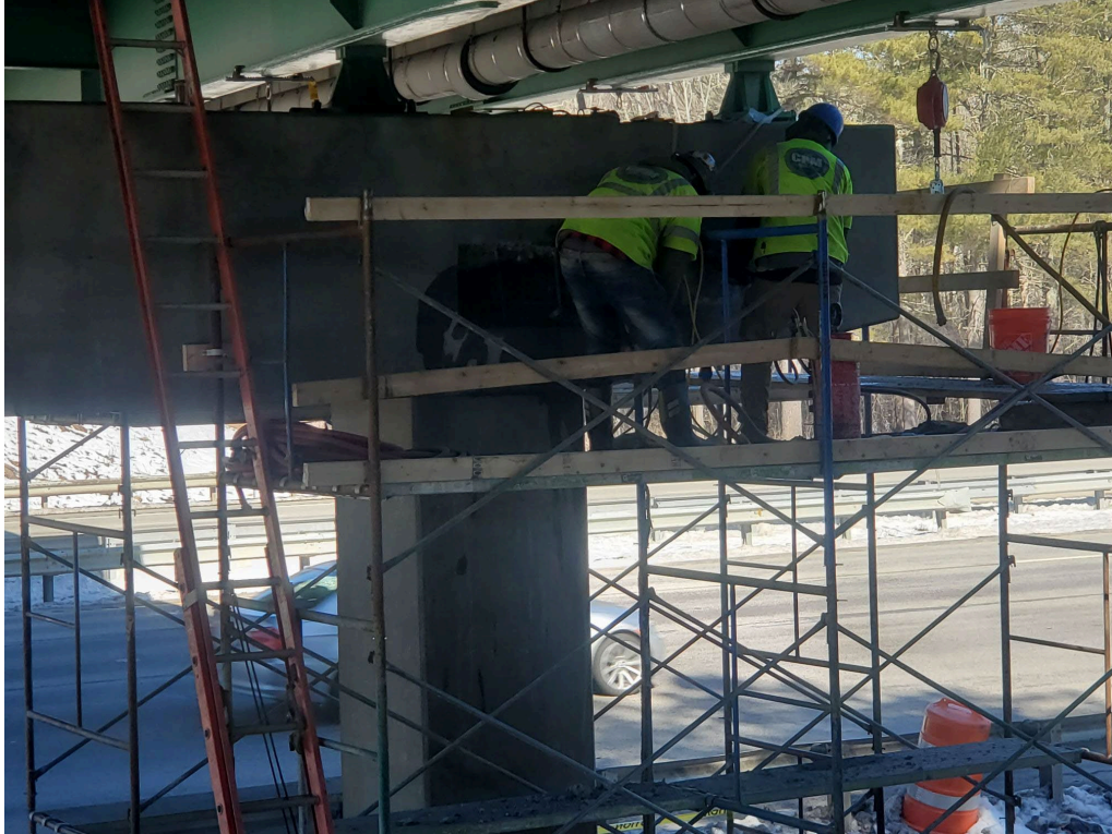
Concrete removals on the east side of Pier 1 at Wilson Road.
