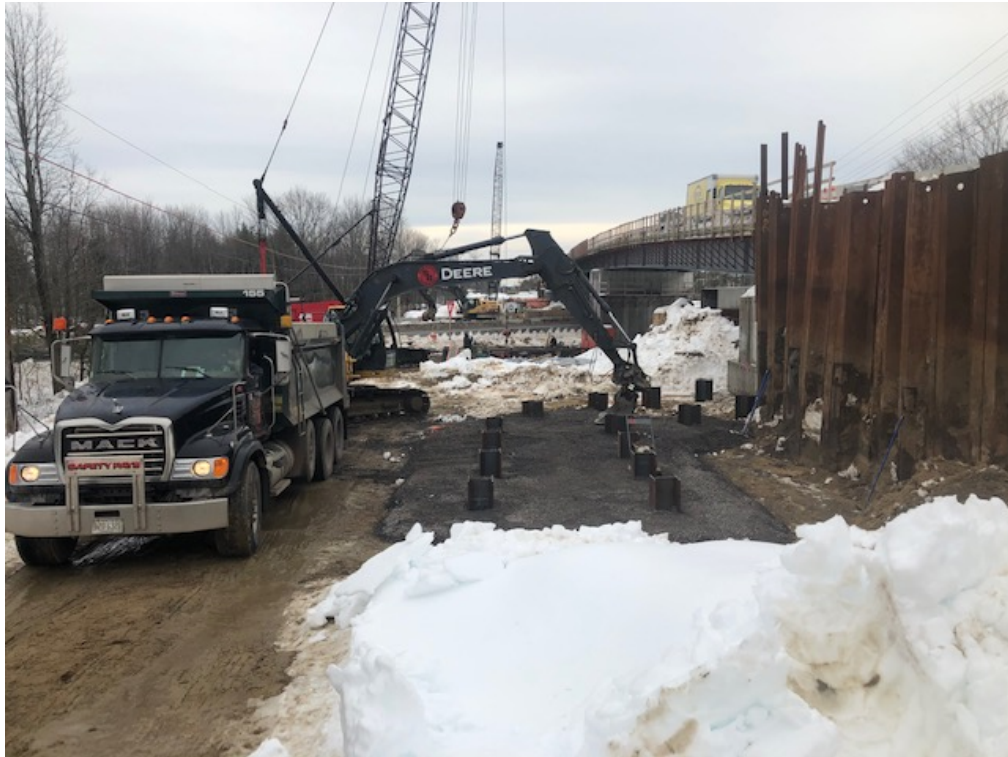
Pile cut off at elevation at abutment 2
