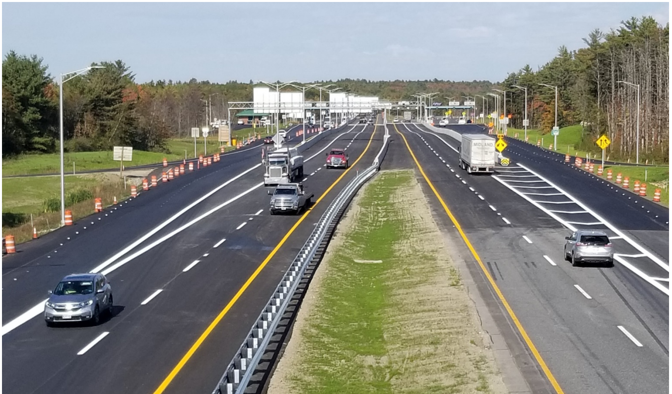
New toll plaza
