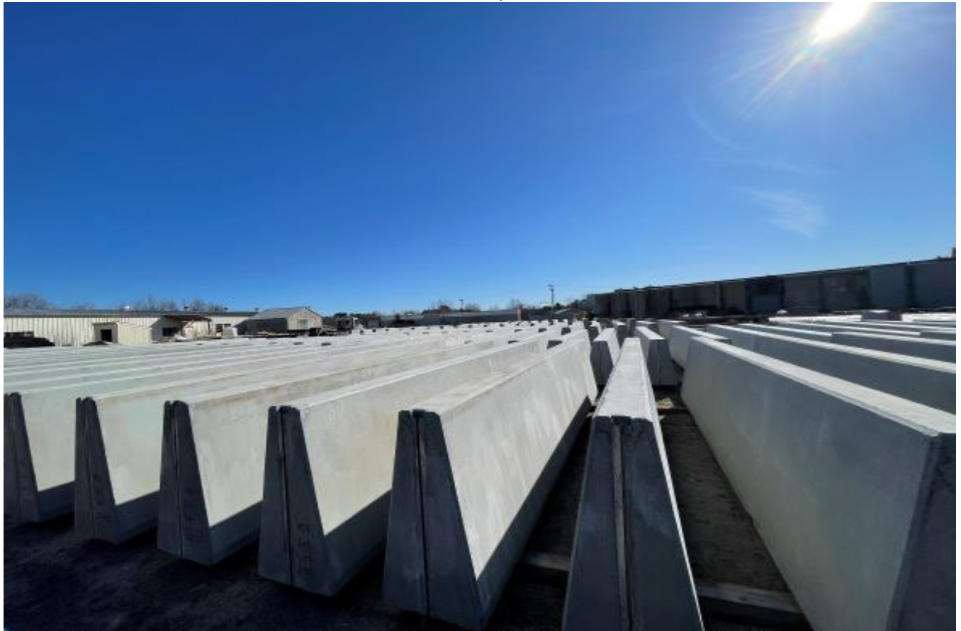
Precast concrete barrier, destined for the York Demolition project, is being stockpiled in the supplier's yard in anticipation for the 2022 construction season
