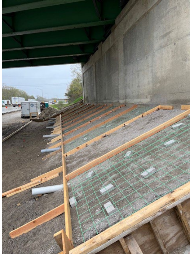
Looking Northbound at the Westbrook Street Slope Protection
