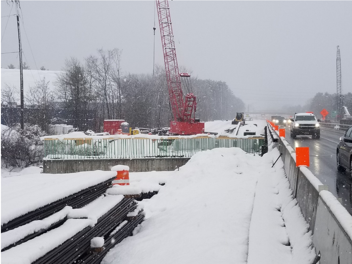
Looking south at Abutment 2 northbound bridge
