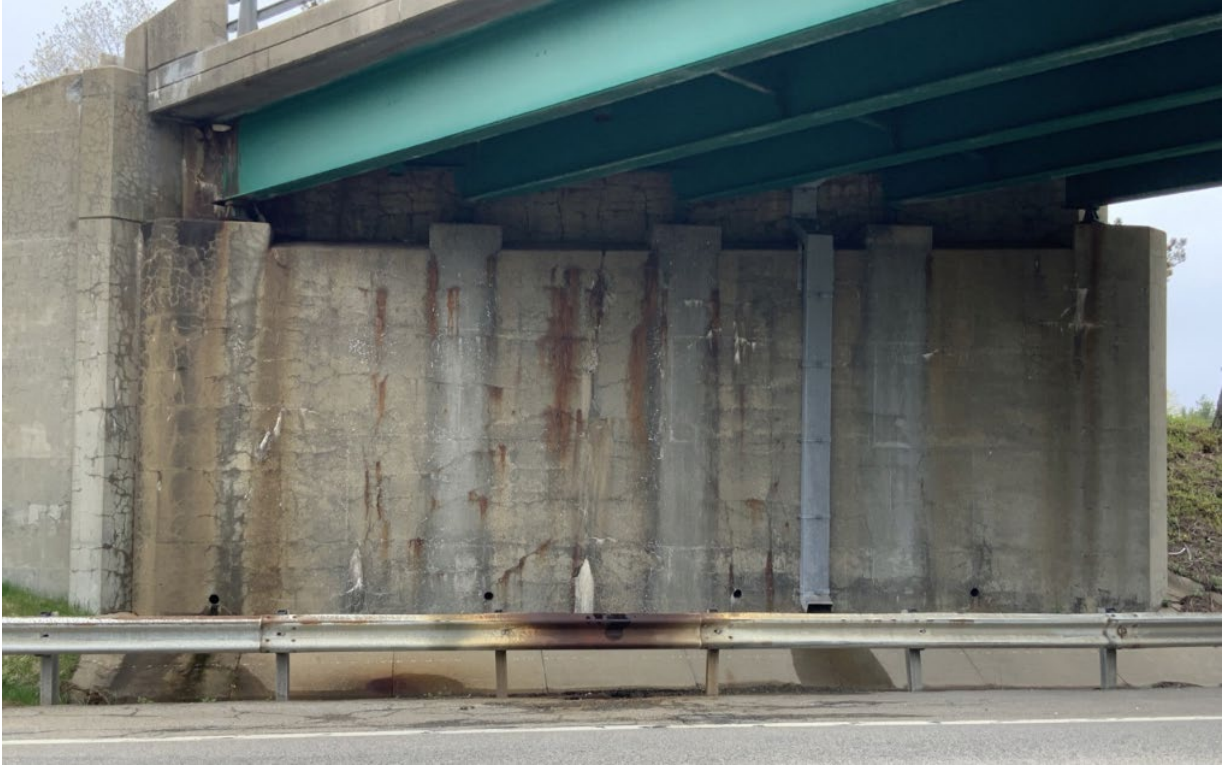
Looking East, Ramp J abutment that will be repaired.
