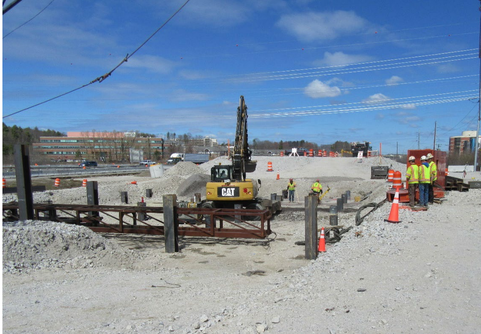
Northbound Toll Plaza – Driving H-pile
