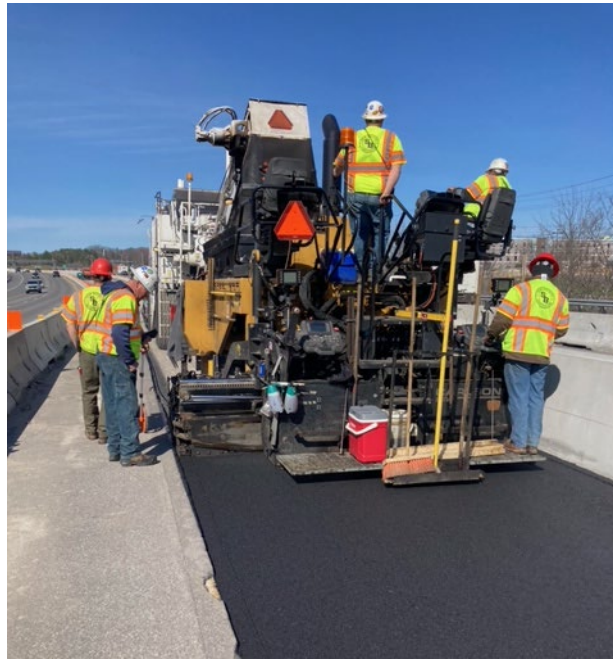
Paving adjacent to the median barrier
