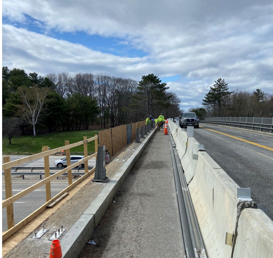
Concrete curb repairs at Wilson Road.
