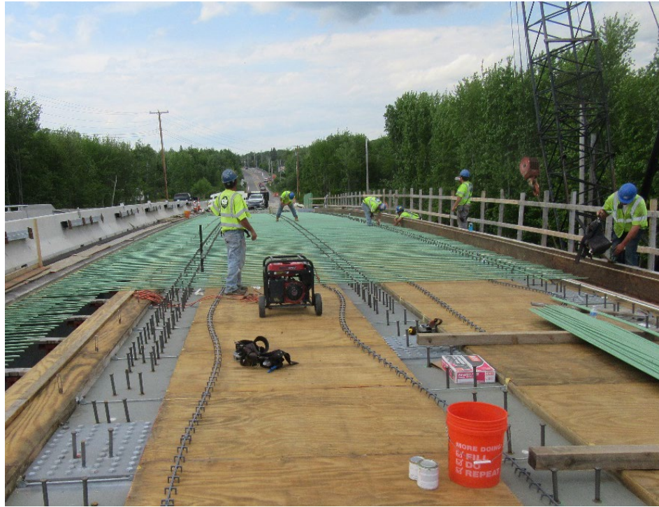
Placing reinforcing steel phase 2 deck placement
