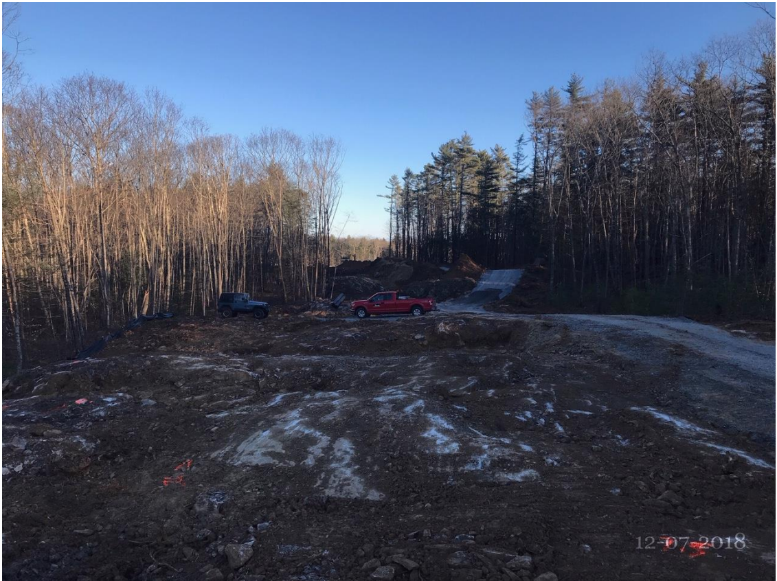
Access Road looking toward Turnpike from Chases Pond Road
