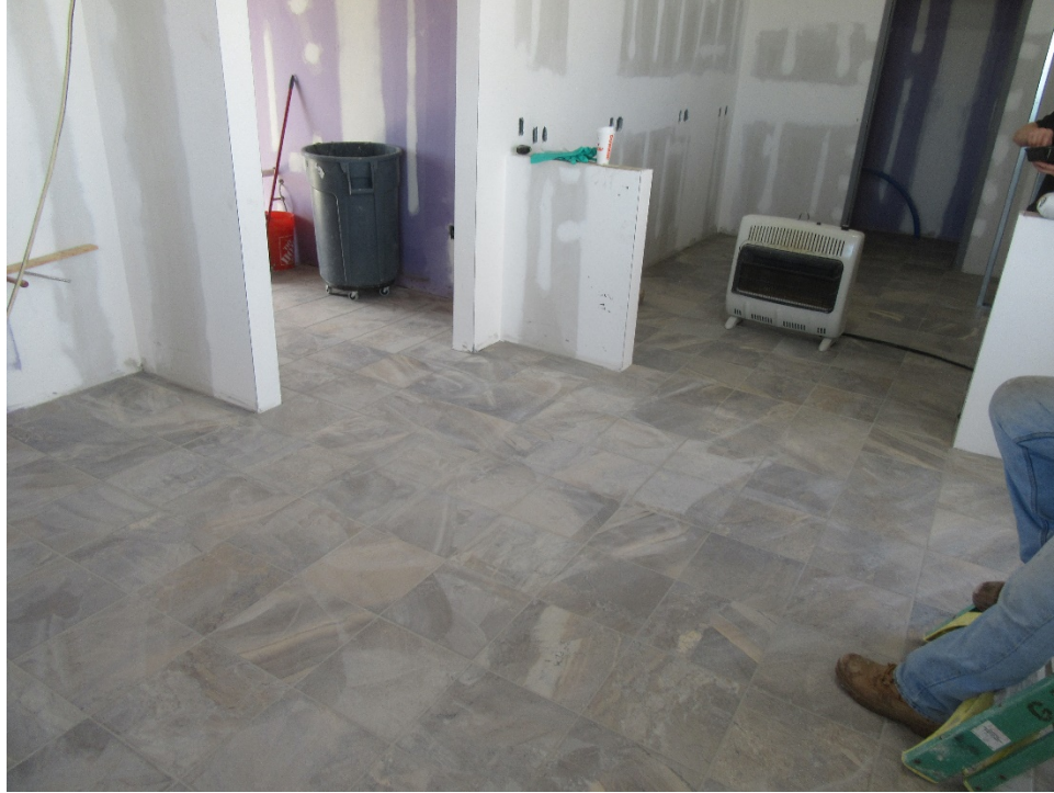
Completing floor tile work in the Northbound Admin building
