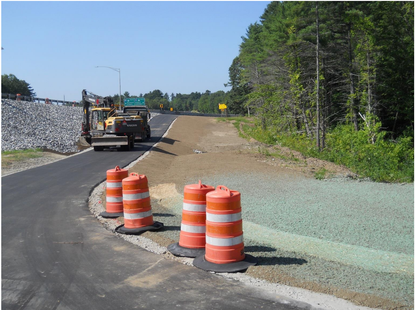
Northbound Emergency Vehicle Access at Exit 52 on-ramp off from Blackstrap Road
