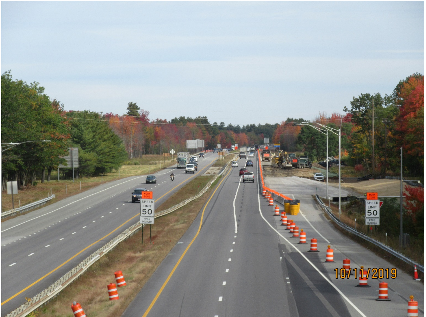
Warren Avenue Bridge looking north
