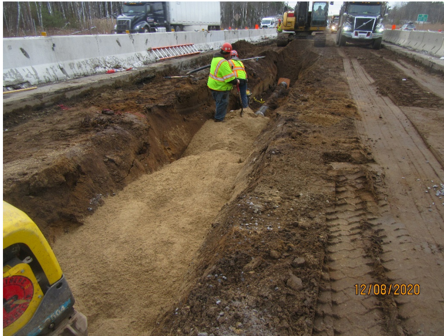
Installing underdrain in the median
