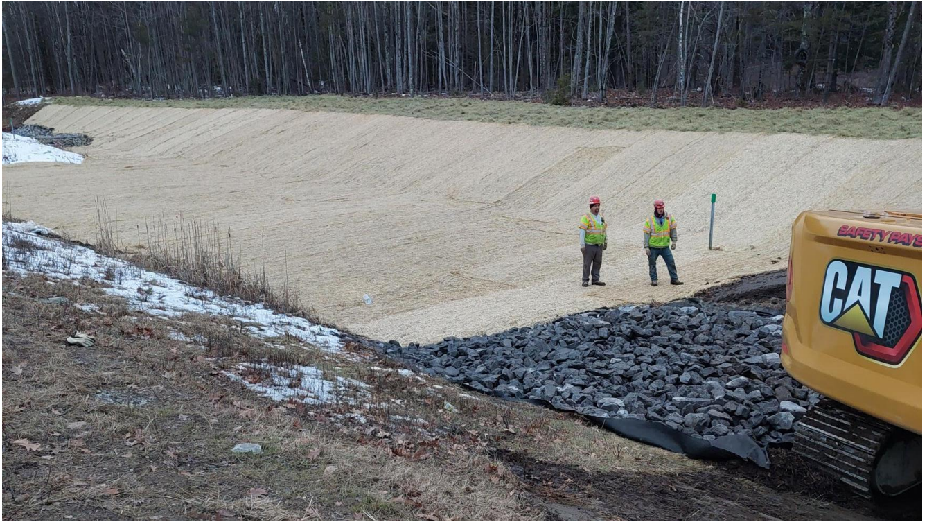
Completed repairs to underdrain soil filter #1 (USF 1).
