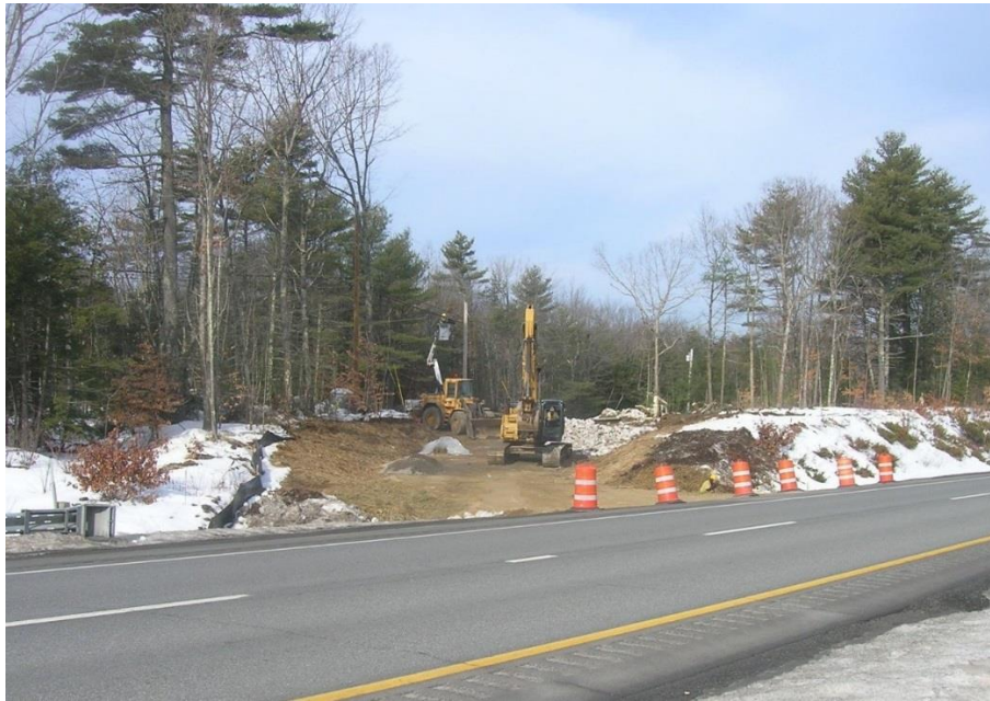
Emergency Access Ramp entrance onto the SB Turnpike lanes
