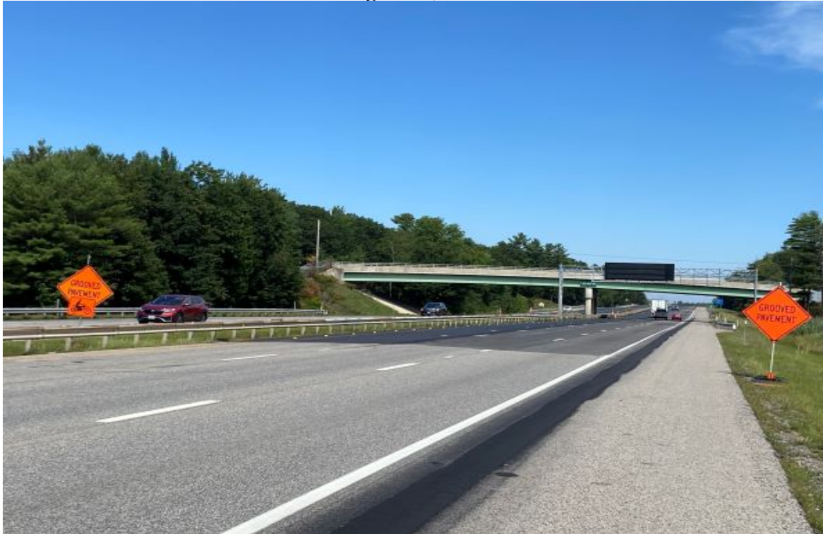
Looking north at the beginning of the project, in Biddeford, (MM30.0 NB).
