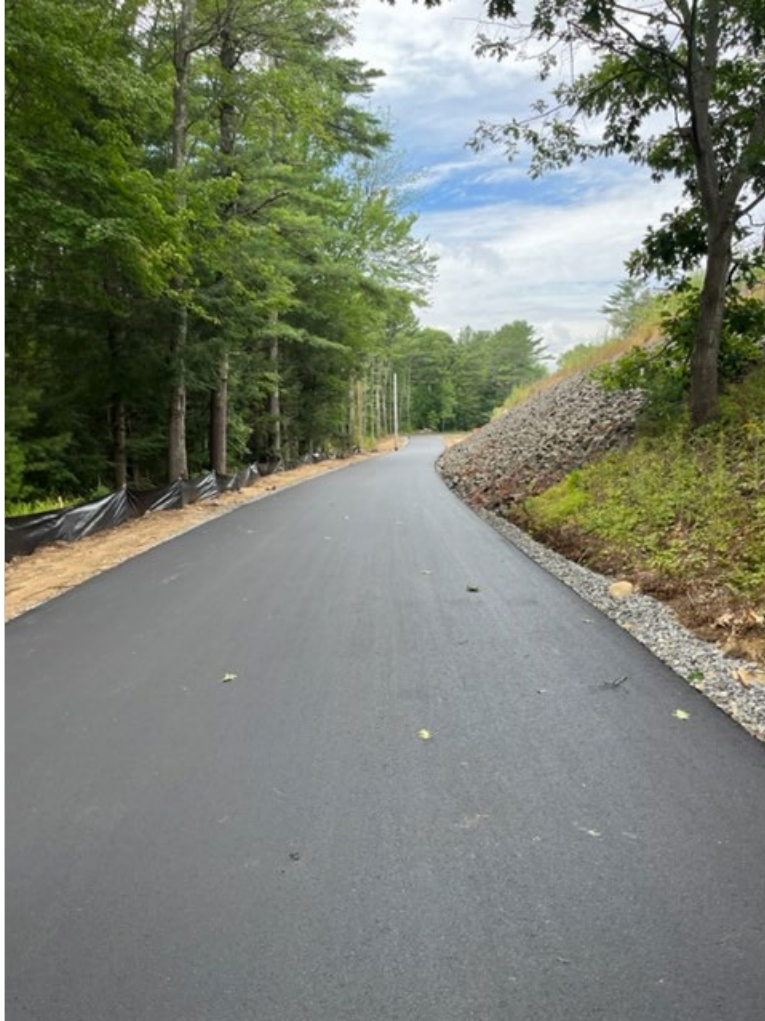
Southbound Emergency Vehicle Ramp
