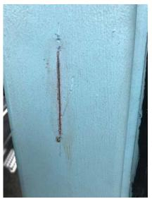
Picture 1: Structural steel supports tested positive for lead paint
