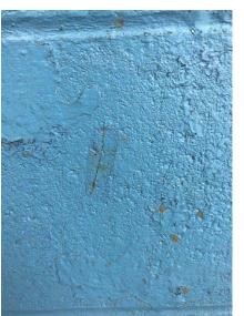
Picture 2: painted cement block at tool booths tested negative for lead paint
