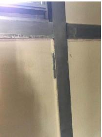
Picture 5: window caulking that tested positive for asbestos, which is attached to the traniste panels
