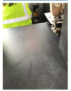
Picture 3: toll booth lab tops are assumed to be asbestos based on previous testing of the materials
