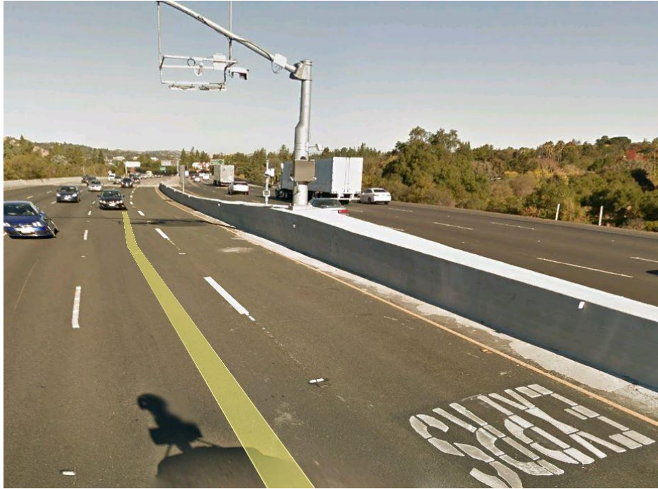
Figure 5 – Open access facility on I-680 in Contra Costa County
