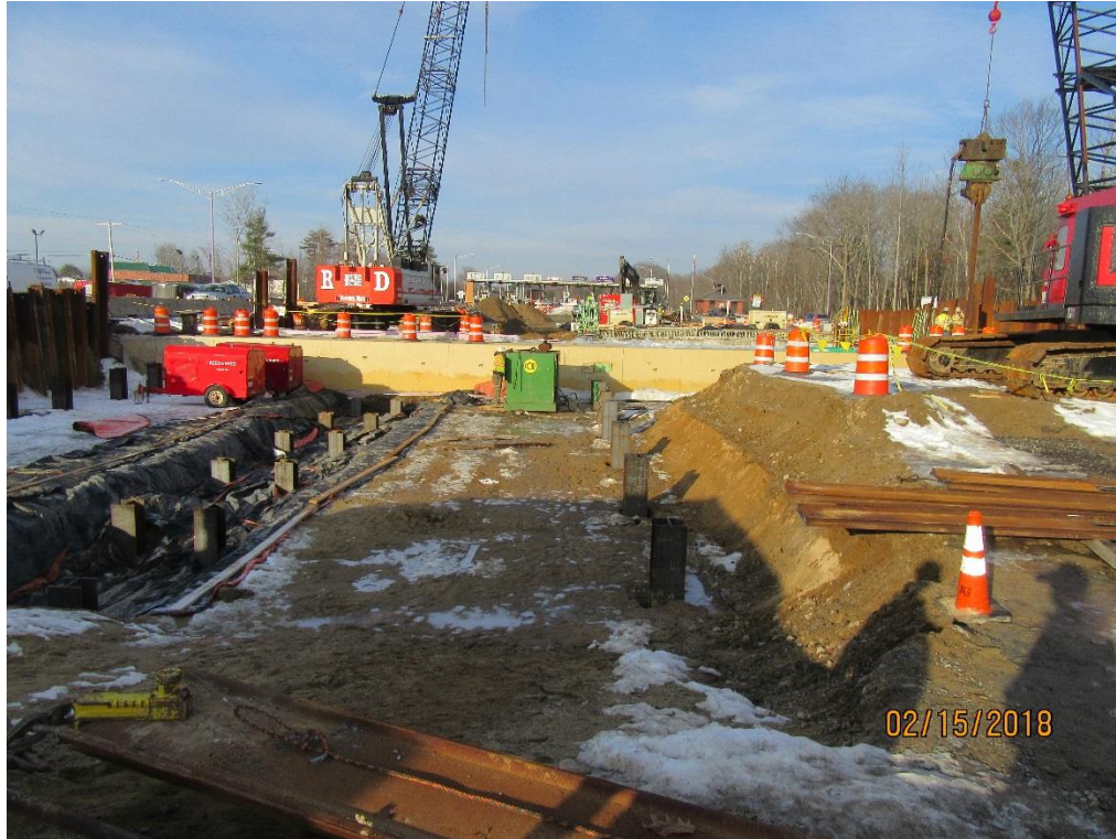
Pile supports for the Northbound Grade Beam supports
