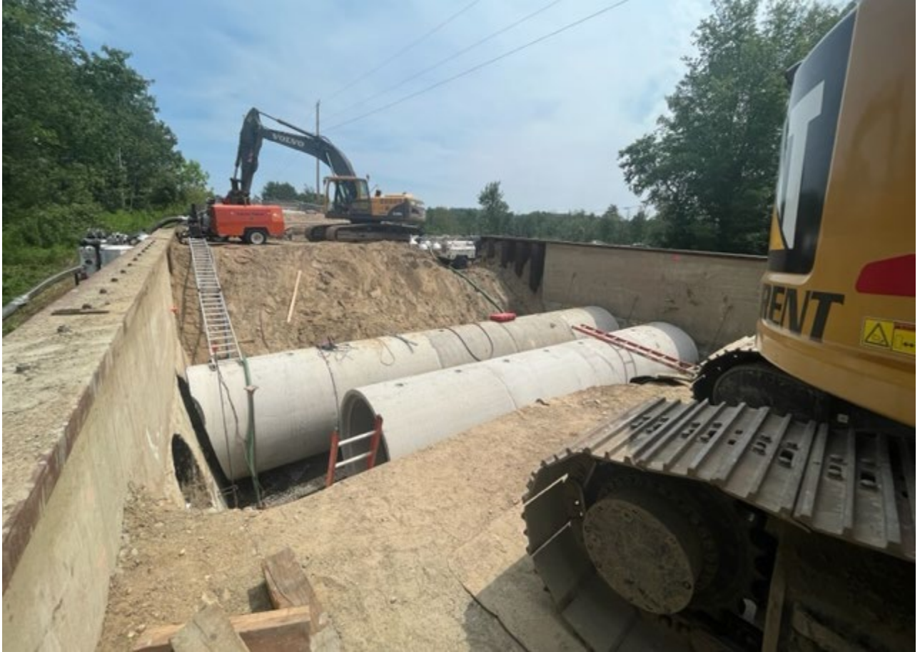
72-inch Concrete Pipes being installed between the existing headwalls
