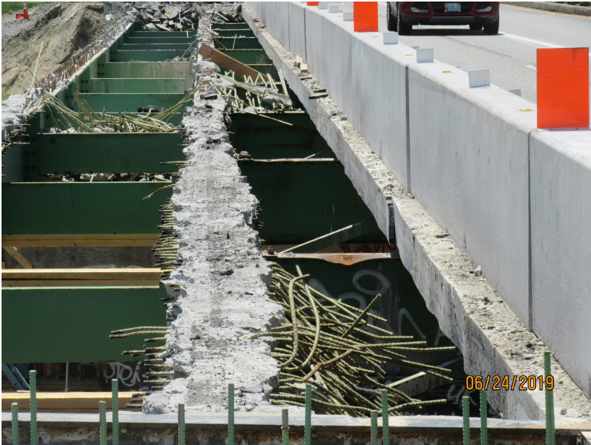
Phase 1 deck demo at MCRR north bound
