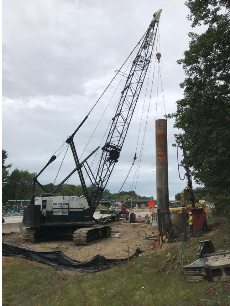
Driving caisson for overhead sign structure foundation
