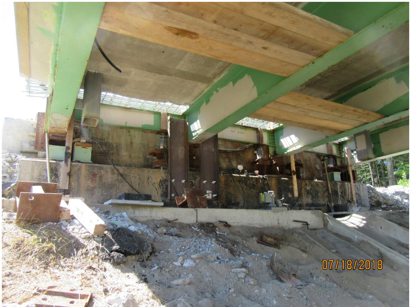
Jacking Weymouth Road Bridge
