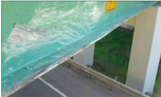
RAMP M BRIDGE, MILE 1.7
