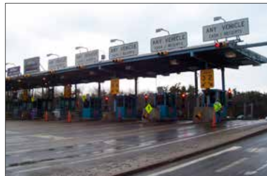
EXISTING YORK TOLL PLAZA - CONSTRUCTED IN 1969
