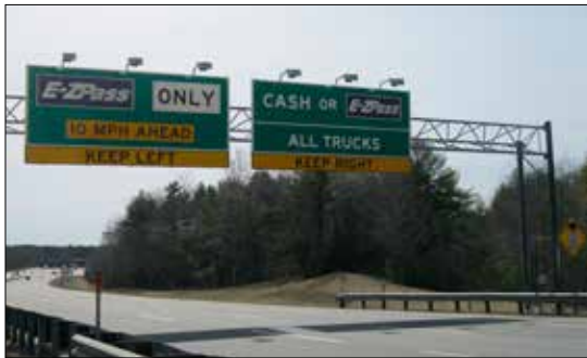
OVERHEAD SIGN BRIDGE MAINLINE SB, MILE 7.8
