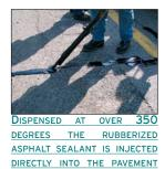
another method of maintaining the pavement in good condition to reduce future maintenance costs. This sealing reduces the water infiltration of the pavement into the subbase helping to extend the life
