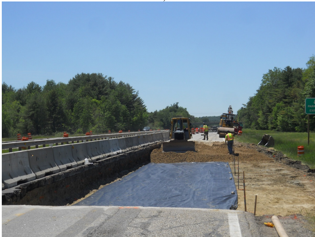
Full depth pavement repair to subgrade
