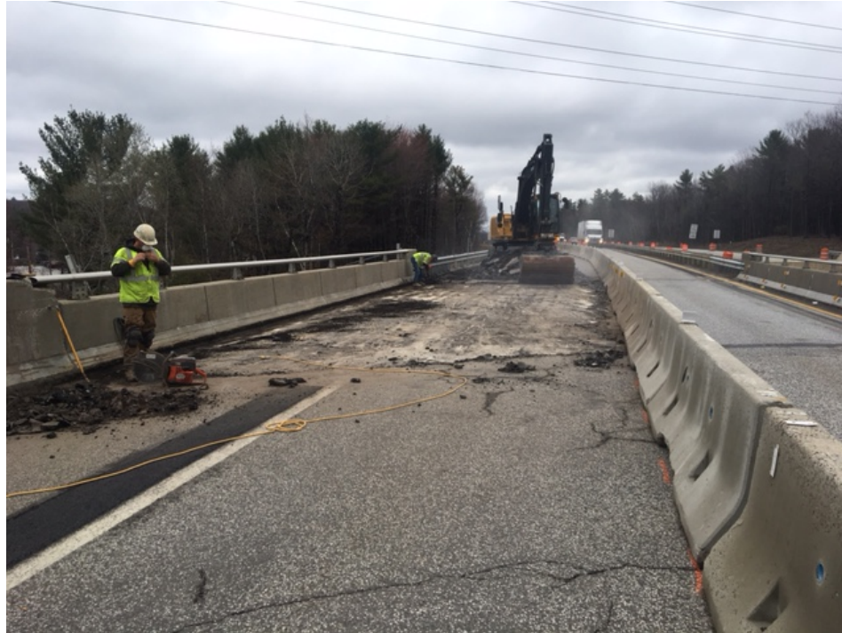
Removing pavement from Ferry Road Bridge
