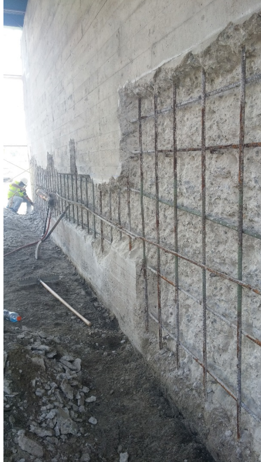
Exit 75 Interchange bridge
