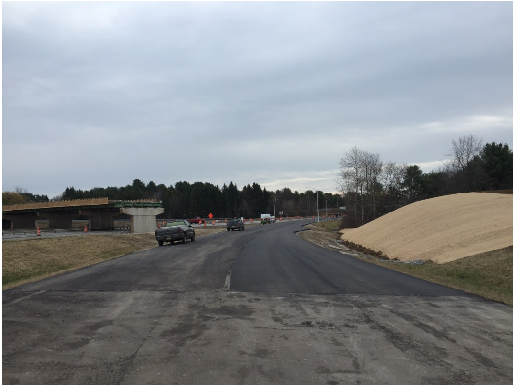
New Southbound on-ramp – portion of interchange bridge removed
