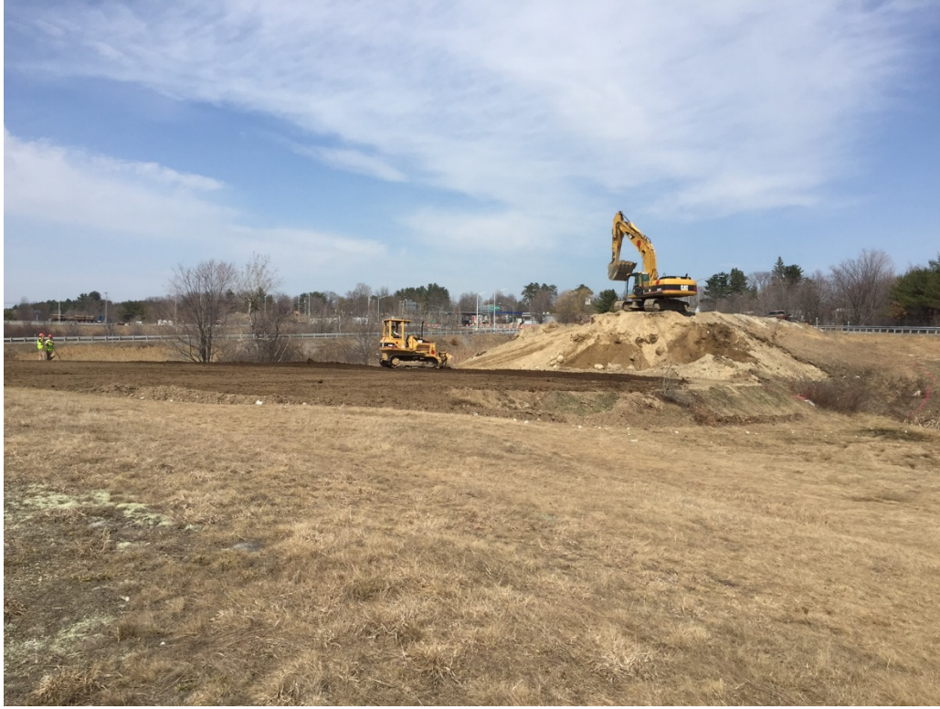
Removing old roadway approach to previous interchange bridge
