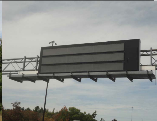
OVERHEAD SIGN STRUCTURE, WALKWAY PLATFORM, AND VMS SUPPORT
