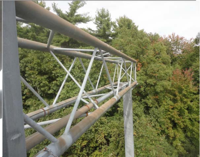
(2) GALVANIZED STEEL CONDUITS FROM VMS TO CONTROLLER CABINET
