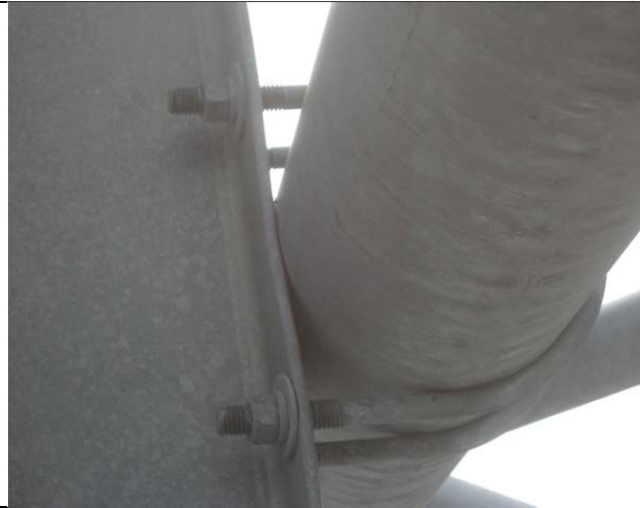
TYPICAL TRUSS MEMBER TO VERTICAL SUPPORT MEMBER (2)U-BOLT CONNECTION
