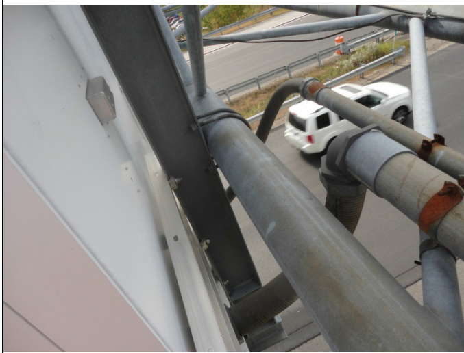
CONDUIT FEED INTO BACK OF VMS. Z-CLIP CONNECTION SIGN TO VERTICAL SUPPORT
