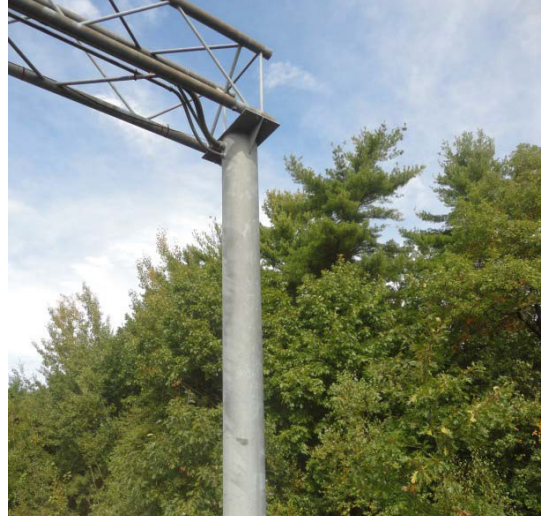
COLUMN CAP PLATE, CONDUIT RUNS FROM VMS TO INSIDE COLUMN (HAND HOLE AT BASE) AND OUT OF FOUNDATION BELOW GRADE TO CONTROLLER CABINET NEARBY
