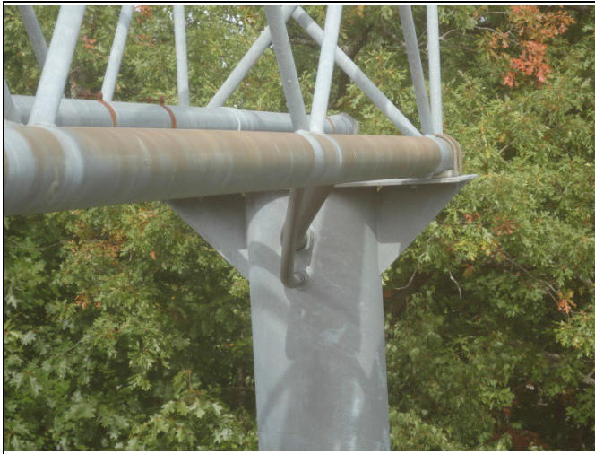
COLUMN CAP TO TRUSS CONNECTION WITH CONDUIT (SIDE SLOPE)
