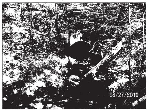
Figure 2 - Same unnamed tributary passing under the Turnpike and through the interchange. This is the inlet located near the park and ride lot on Alfred Plourde Parkway between the northbound ramps and the Turnpike. This pipe flows under the Turnpike and into the southbound ramp in-fields.
