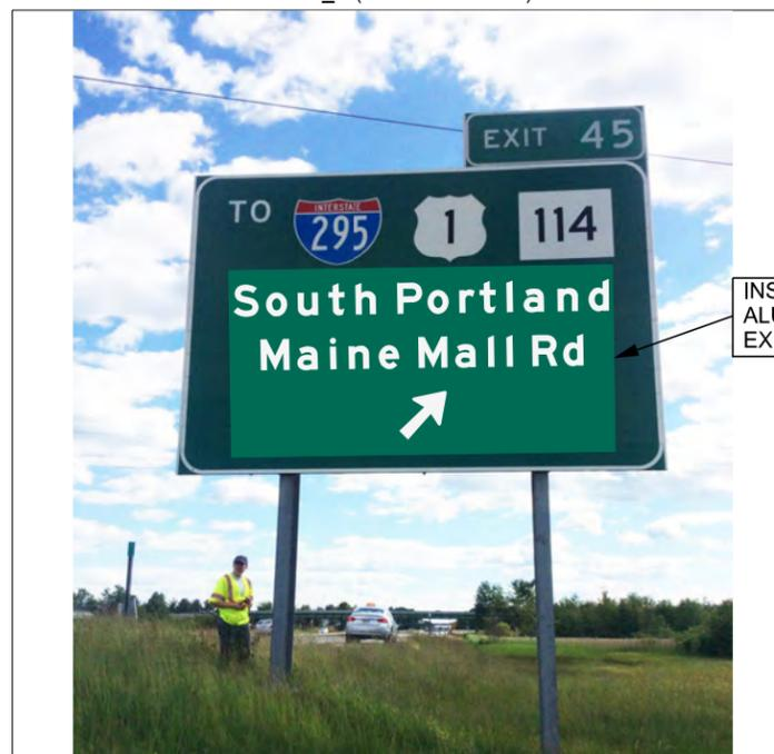
INSTALL NEW SHEET ALUMINUM OVERLAY OL-2 ON EXISTING SIGN
